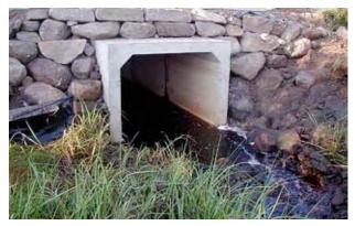
New box culvert that allows full tidal flushing (MA CZM photo)
