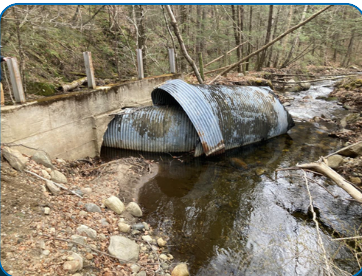
Culvert removal project located on Ratlum Brook. The culvert has been completely washed out and the stream diverted to the old Town road bed.
